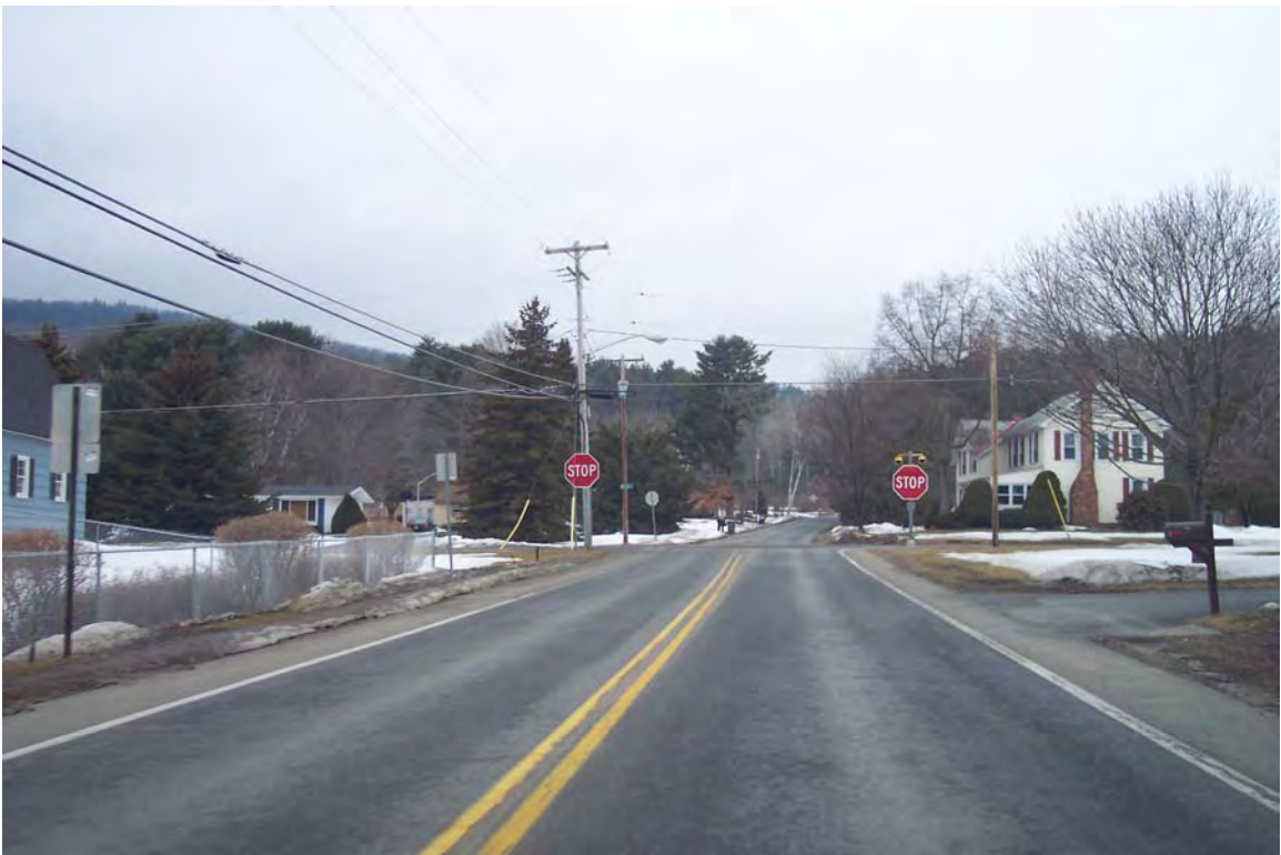
Aviation Road looking west at the West Mountain Road Intersection
