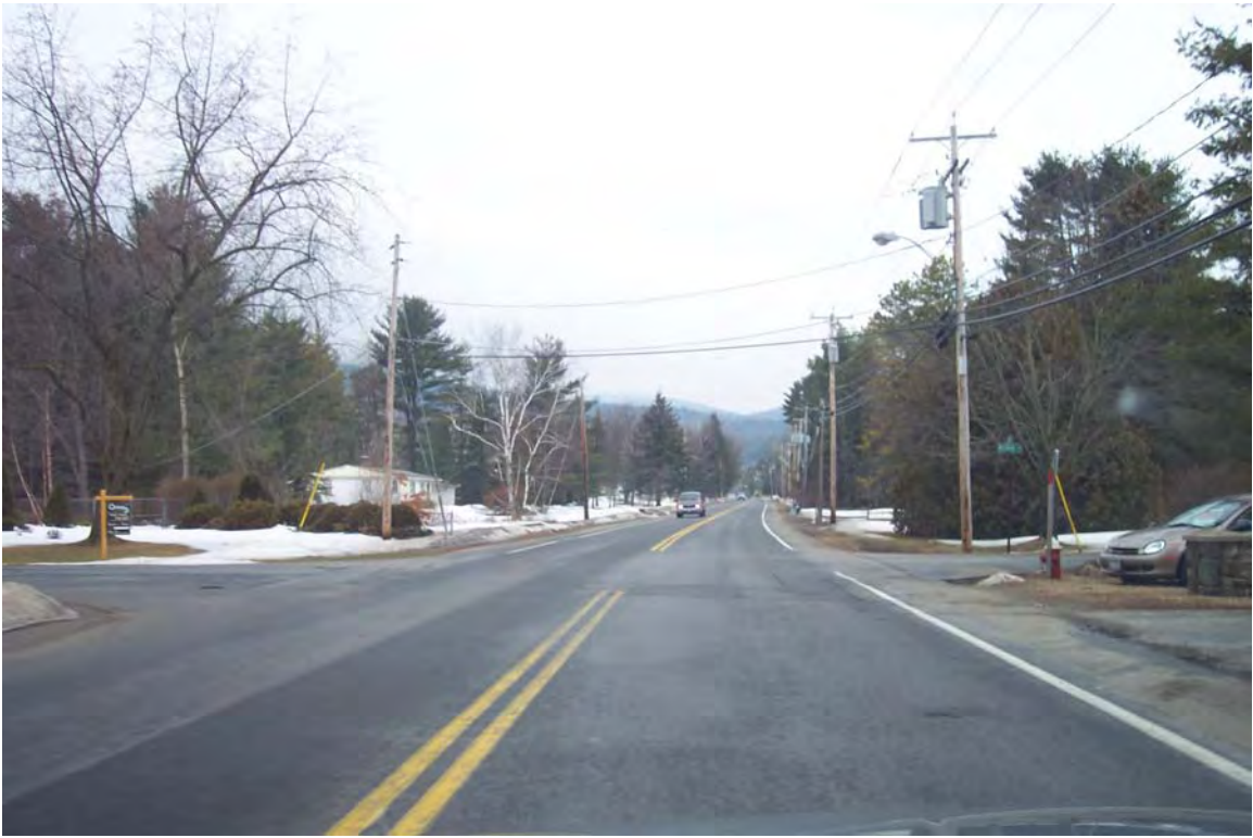
Aviation Road looking west toward the Westmore Avenue/Buena Vista Avenue Intersection
