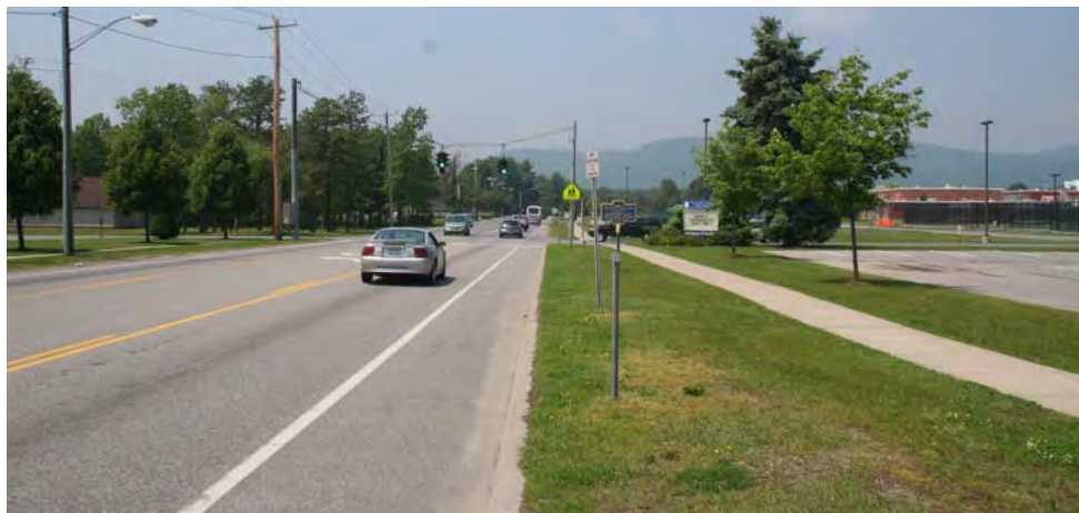
A right turn only lane would be constructed between the existing travel lane(s) and school parking lot. This potential capacity expansion would need to be compatible with school improvement plans and must ensure that sidewalk(s) be replaced should the existing concrete be removed.
