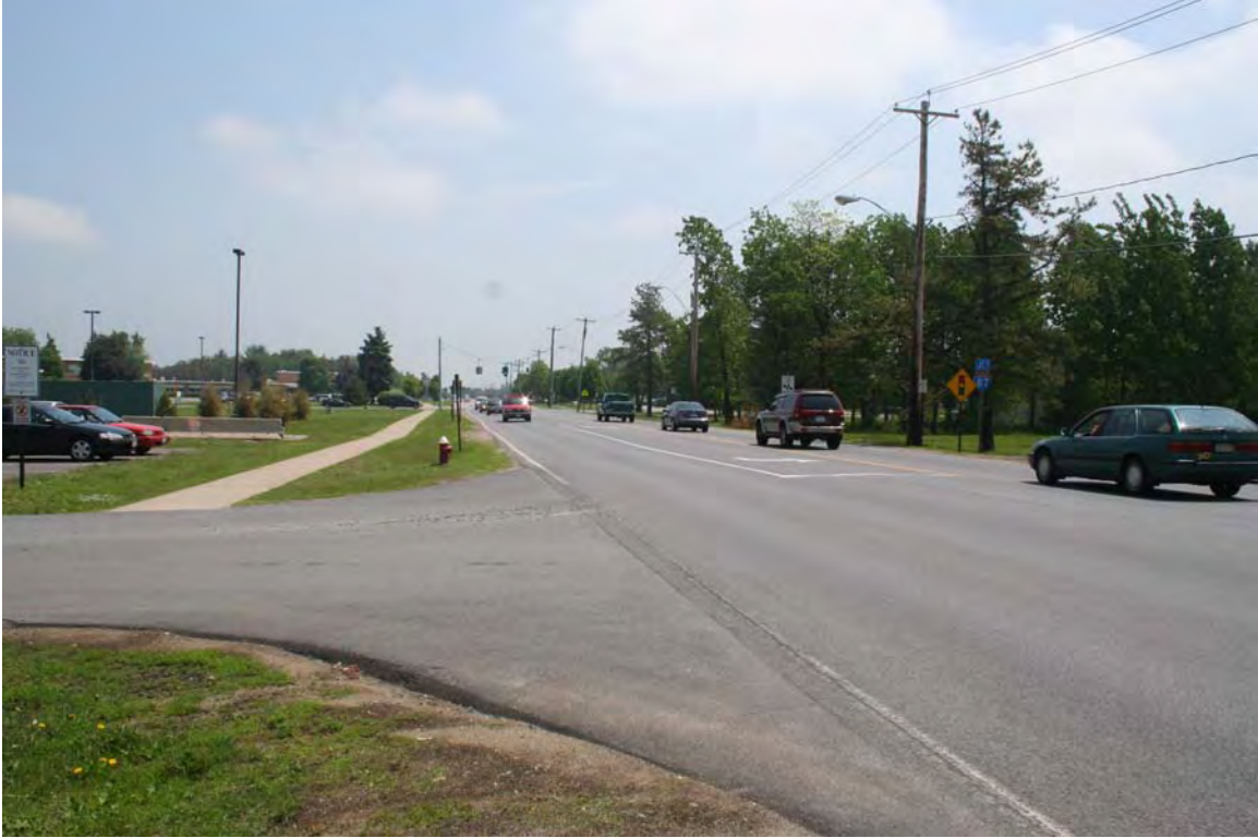
Aviation Road looking east at the Queensbury High School eastern driveway
