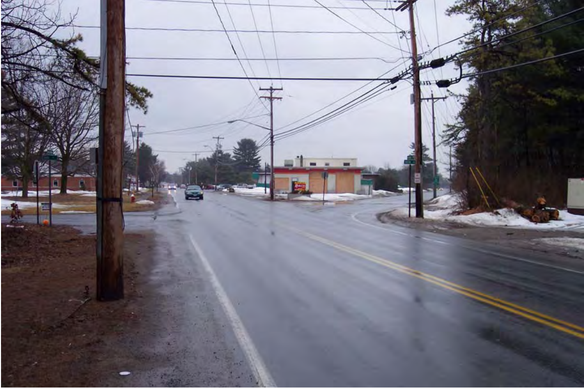
Aviation Road looking east at the intersection of Dixon Road/Farr Lane
