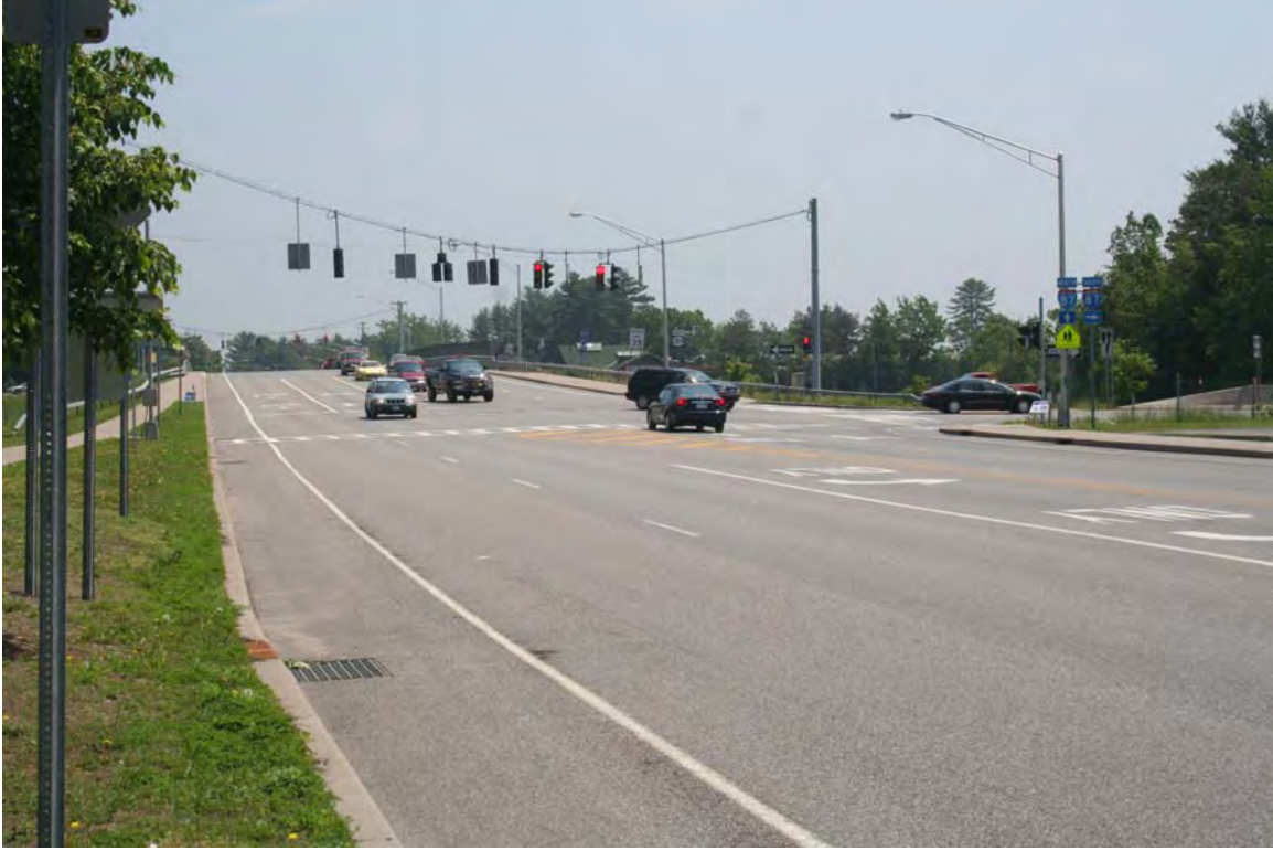
Aviation Road looking east at the Aviation Road/Burke Drive Intersection and I-87 overpass
